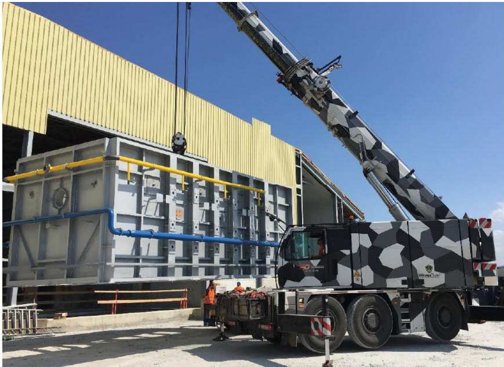
Installation of the furnace 7 x 1,8 x 3,5 m
